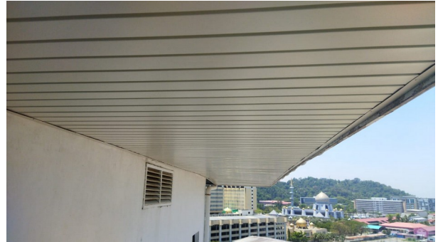
Ceiling work photographed during the project.
