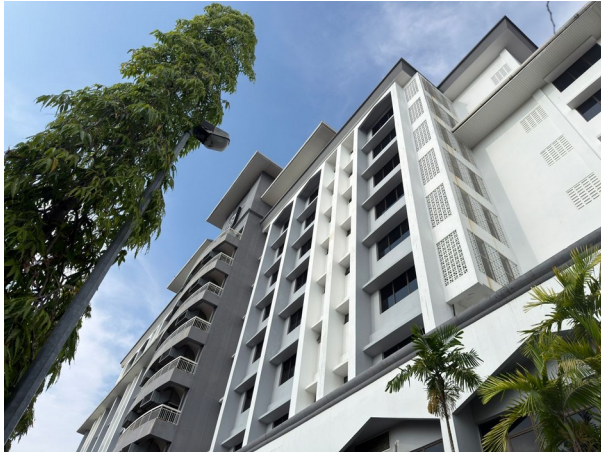
Raia Hotel: completed-work photograph in the final report.
