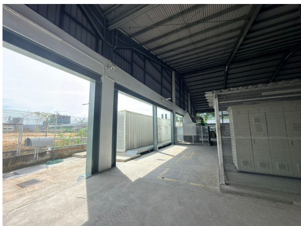
MSC Kolombong: completed-work photograph in the final report.
