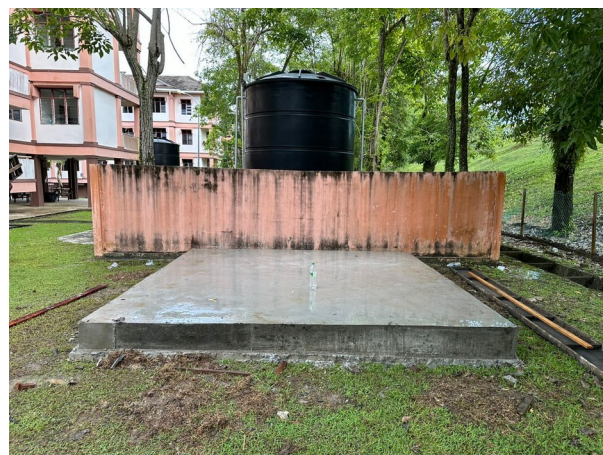
Concrete base works photographed during the project.
