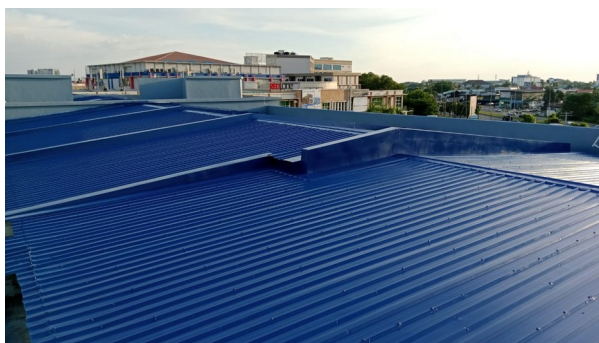
Roof finish shown in the project report.
