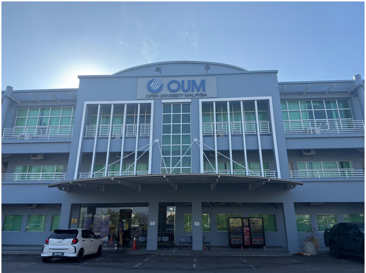
OUM Learning Centre, Kota Kinabalu — a PA refurbishment project.
